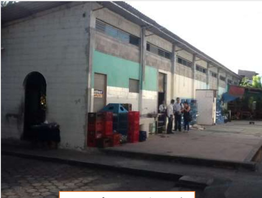
Area of construction and restoration for the classrooms
